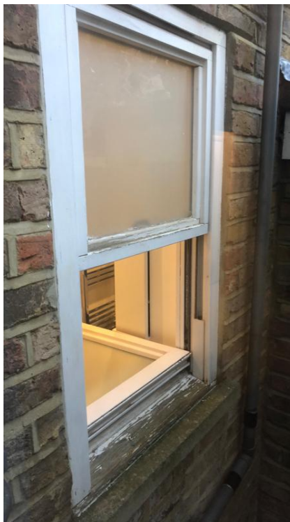
Weathering was noted to the bathroom window and window frame
