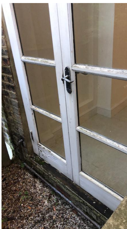
Weathering was noted to the rear bedroom doors and doorframe
