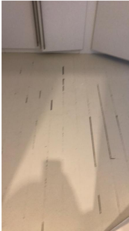
Gaps were noted between the floorboards throughout the property
