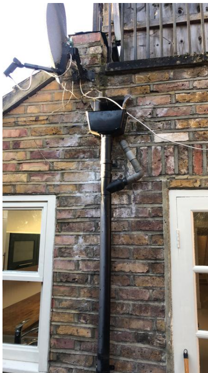
Efflorescence was noted to the rear elevation
