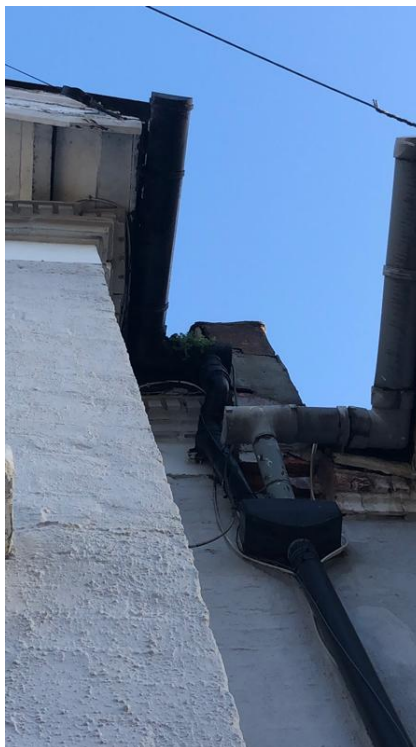
Vegetation was noted in the front gutter
