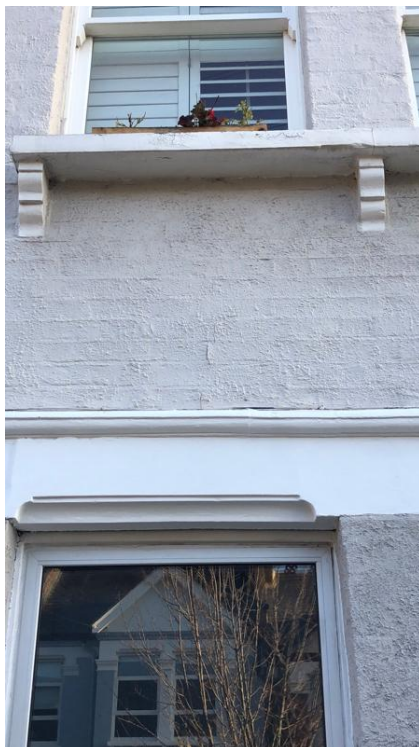
Settlement cracking was noted to the front elevation
