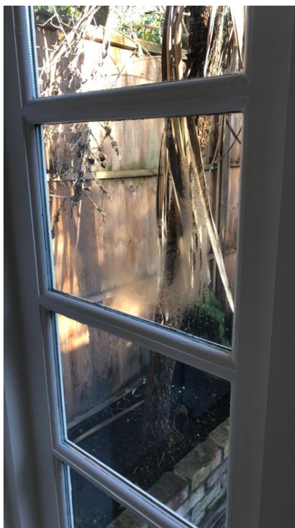
A failed glazing unit was noted to the rear window
