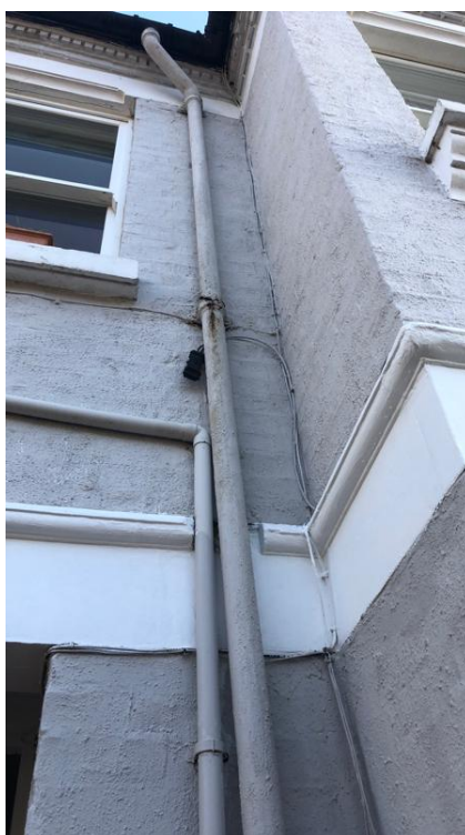
Deterioration was noted to the joints of the gutters and downpipes
