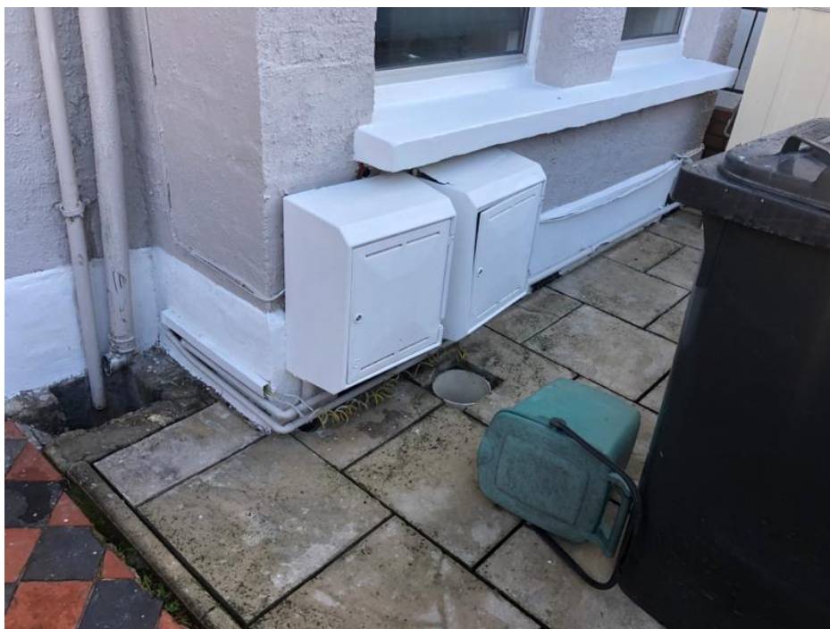
Render upstand to base of wall
