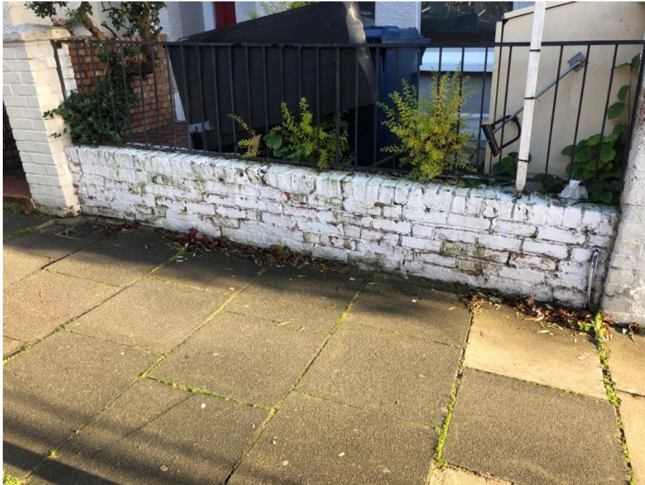
Spalled bricks were noted to the front boundary wall
